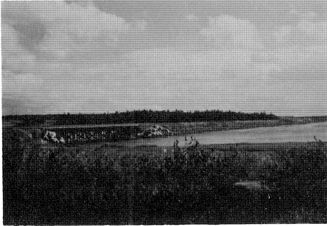
Railway Bridge at Lawrencetown Lake
